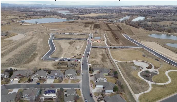
Overall (View: North)
