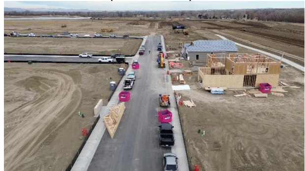
Colorado River Drive (View: North)
