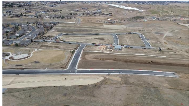
Phase I & II (View: West)
