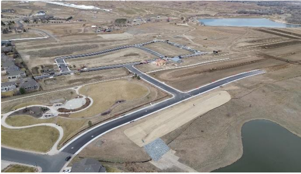
Overall (View: Northwest)
